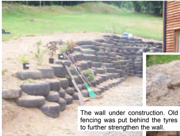
The wall under construction. Old fencing was put behind the tyres to further strengthen the wall.
